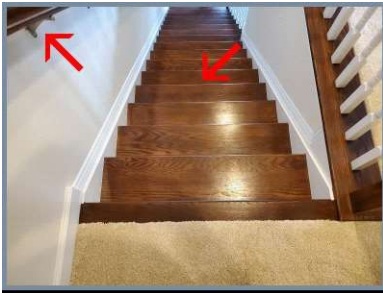
Interior stairs and handrails
