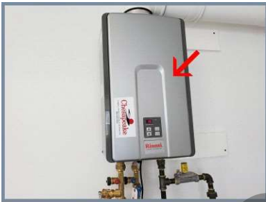
On demand water heater in garage.
