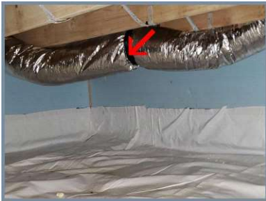
Ductwork in crawlspace.
