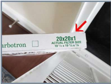
Air filter in front foyer.
