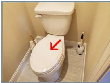
Loose toilet in master bathroom.
