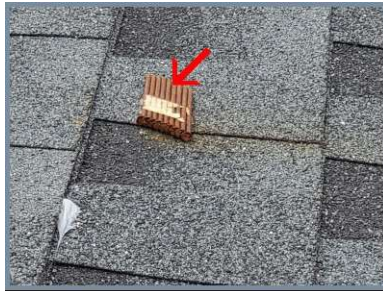
Nails on roof.
