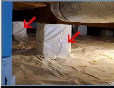
Concrete piers in crawlspace.
