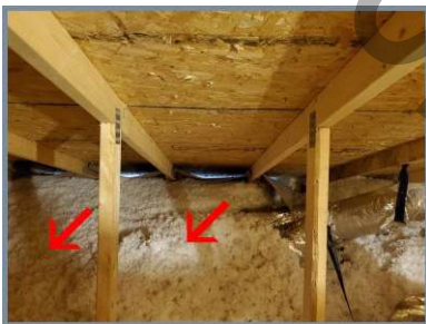
Blown fiberglass insulation.
