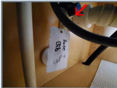
Shutoff valve for left side hose bib.
