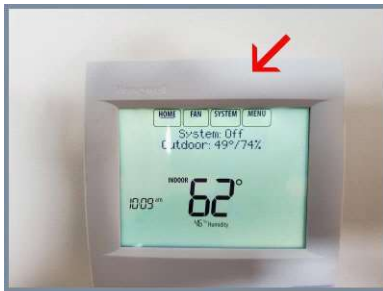
Thermostat at 2nd floor hall bedroom.
