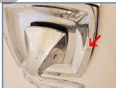
Tub faucet in 2nd floor hall bedroom bath.
