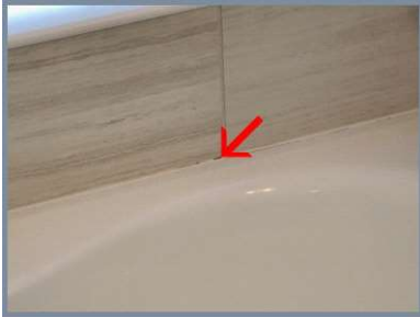
Missing caulk at jetted tub / master bath
