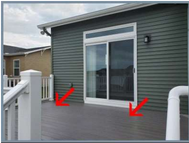
Composite deck at rear.
