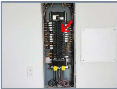
Main electrical panel in garage.
