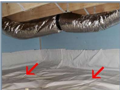
Vapor barrier at floor of crawlspace.
