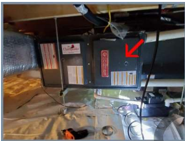
Furnace in crawlspace.
