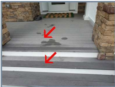
Exterior steps and front porch.
