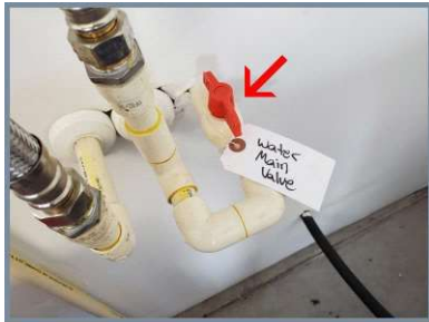
Main water shutoff valve.
