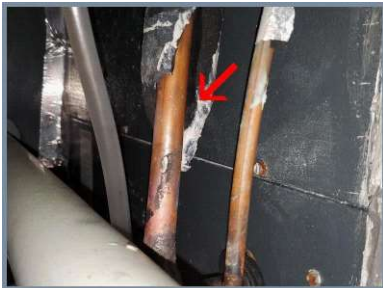
Missing/damaged insulation.
