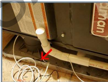
Overflow pan switch at attic unit.
