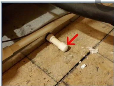
Incomplete secondary condensate drain.
