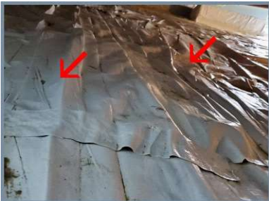
Moisture at crawlspace vapor barrier.
