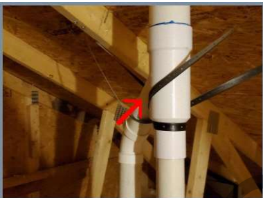
Gas furnace flue.
