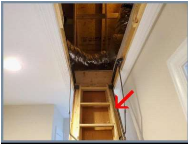
Attic pull down stairs.
