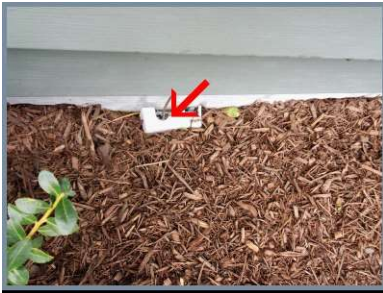
Exterior grounding system.
