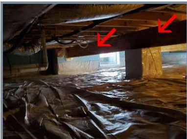
Main beam in crawlspace.
