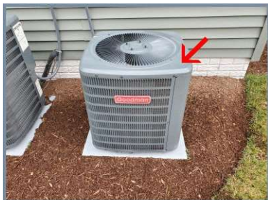
Outdoor HVAC unit for 2nd floor.
