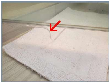
Damaged shower door sweep.
