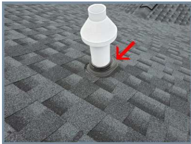
Roof flashings.
