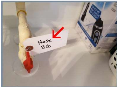
Shutoff valve for right side hose bib.
