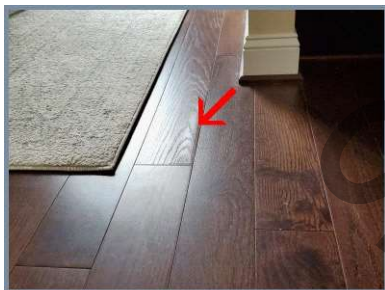
Uneven flooring in dining room.
