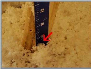
Depth of insulation.
