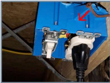
Missing cover plate in crawlspace.
