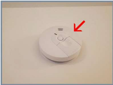
Combo Smoke/Carbon Monoxide detector.
