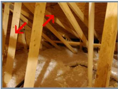
Trusses and osb sheathing.
