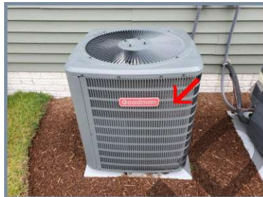
Outdoor HVAC unit for main level
