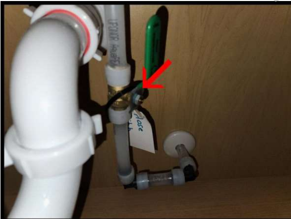
Exterior hose bib shutoff valves.
