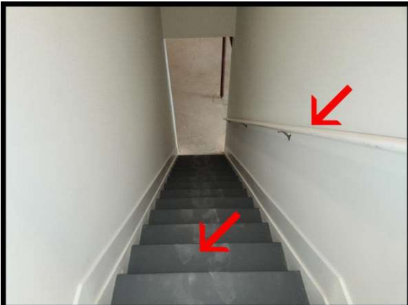
Basement stairs & handrails.
