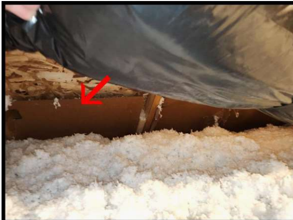
Attic soffit vents.
