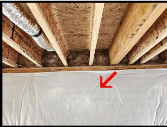
Foundation wall insulation.
