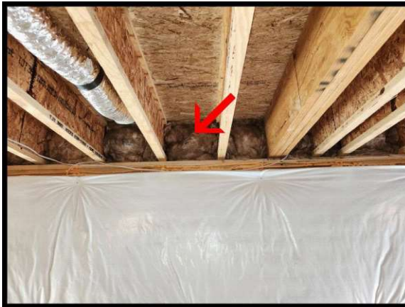
Rim joist insulation.
