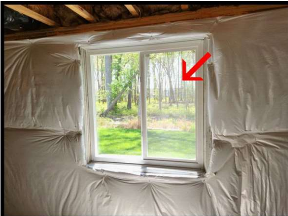
Basement egress window.
