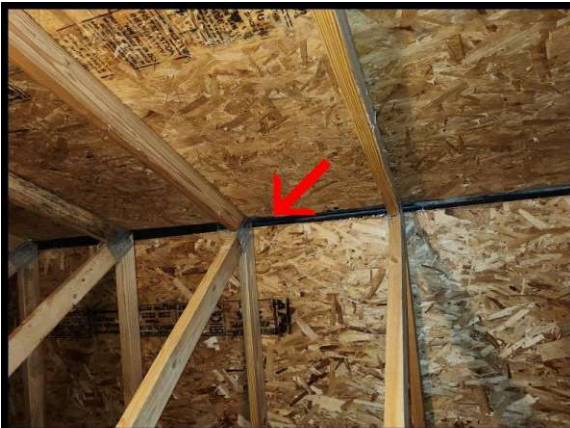
Attic ridge vents.
