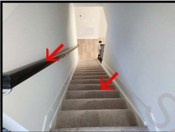
Interior stairs & handrails.
